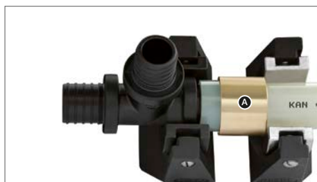
Installation of PPSU elbows and tees \varnothing 25 \times 3,5
